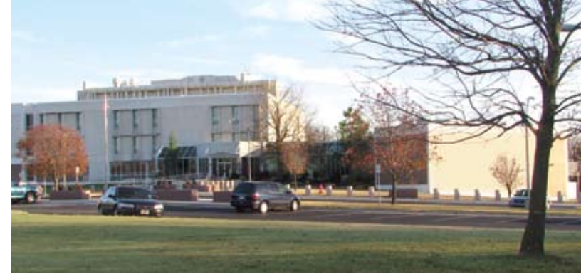
Robert S. Kerr Environmental Research Center, Ada, OK
