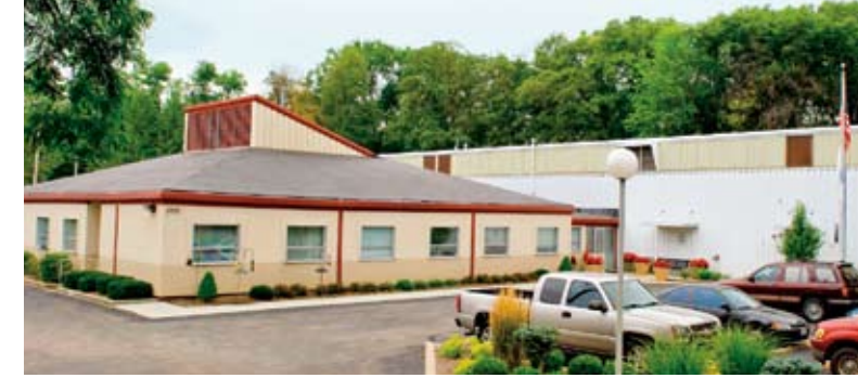
EPA Center Hill Research Facility, Cincinnati, OH
