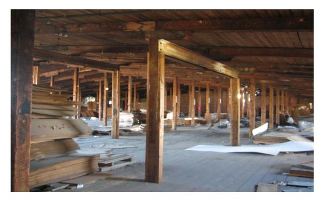
**Photograph No. 1:** Thornhill 7A (upstairs)—view of 6"x 6" timber column structure
