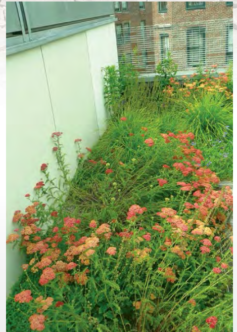
Developers of Philadelphia's Thin Flats condominiums added green roofs that capture rain water and provide private green space, complete with rooftop patios, for each unit.
