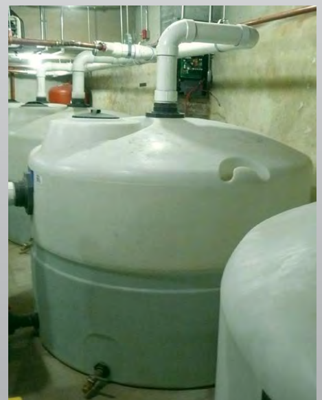
Cisterns operate as part of a rainwater harvesting system in Philadelphia that collects roof runoff for uses such as landscape irrigation or water reuse.
