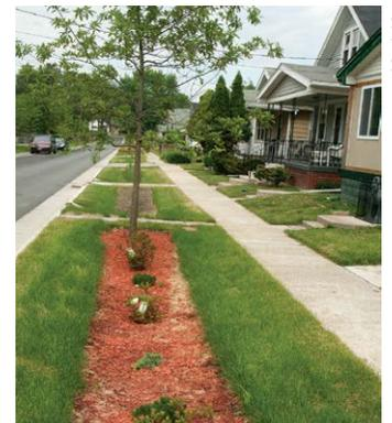
Stormwater from the road and sidewalks flows into this bioretention system on Maywood Avenue in Toledo.
