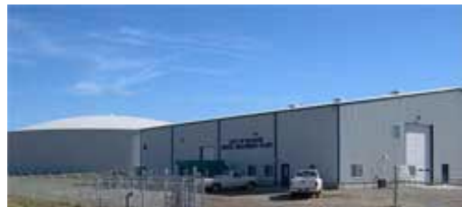
McCook's new water treatment facility including a new 4 MG water storage tank.
