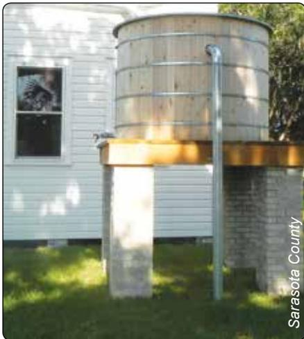
Cisterns provide a higher water-holding capacity than a typical rain barrel. They can be outfitted with filters or other water purification methods when the water is meant for use inside the home.
