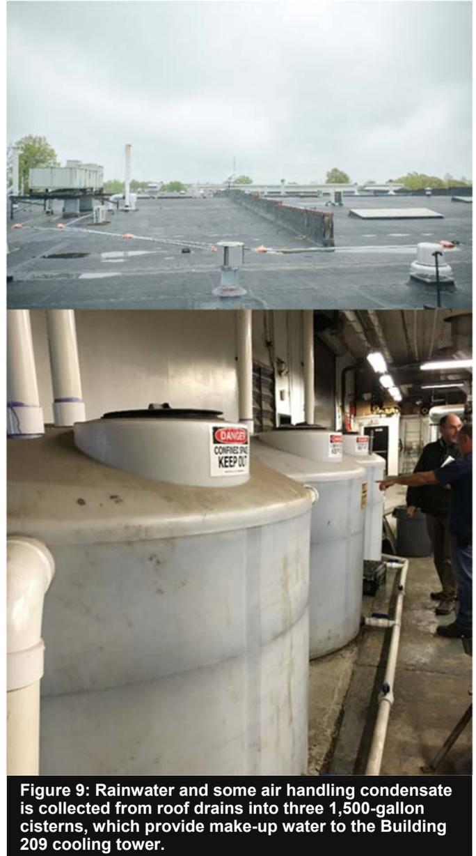
**Figure 9: Rainwater and some air handling condensate is collected from roof drains into three 1,500-gallon cisterns, which provide make-up water to the Building 209 cooling tower.**
