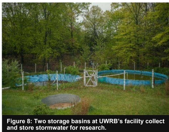
**Figure 8: Two storage basins at UWRB's facility collect and store stormwater for research.**
