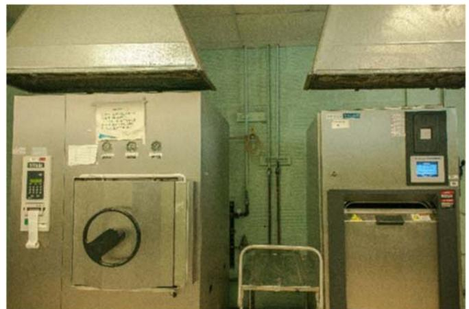
**Figure 6: EEC operates two steam sterilizers, which both have tempering water control systems to eliminate continuous flow of tempering water.**
