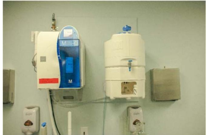
**Figure 7: EEC has multiple small RO systems that provide purified water in individual laboratories.**
