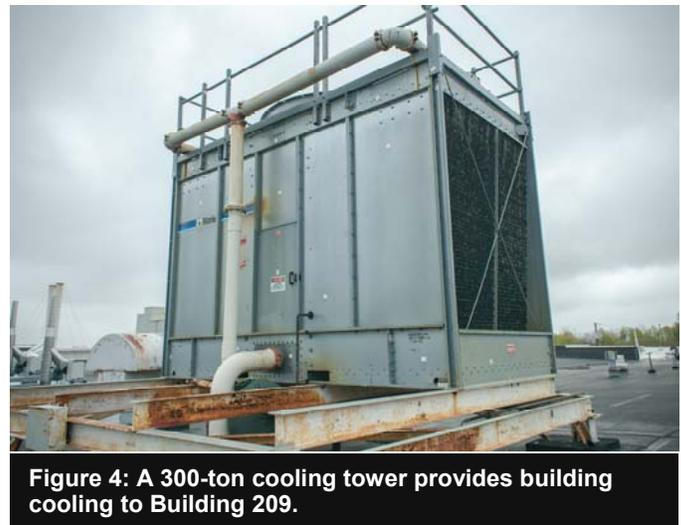
**Figure 4: A 300-ton cooling tower provides building cooling to Building 209.**
