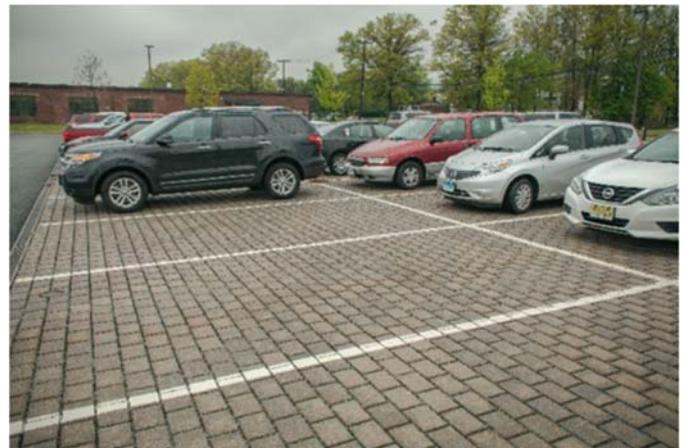
**Figure 10: Three types of permeable pavement are installed in the main employee parking area at EEC.**
