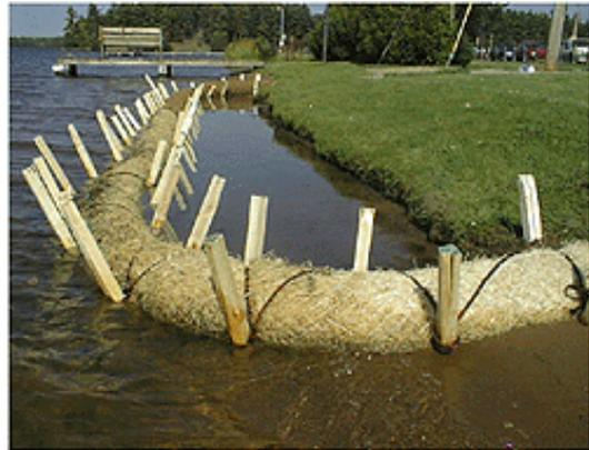
Figure 7.12 Coconut Fiber Roll (Montgomery Watson, 2001)
