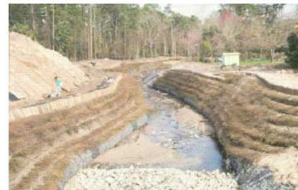
Figure 7.32 VRSS Structure After Construction (Sotir and Fischenich, 2003)
