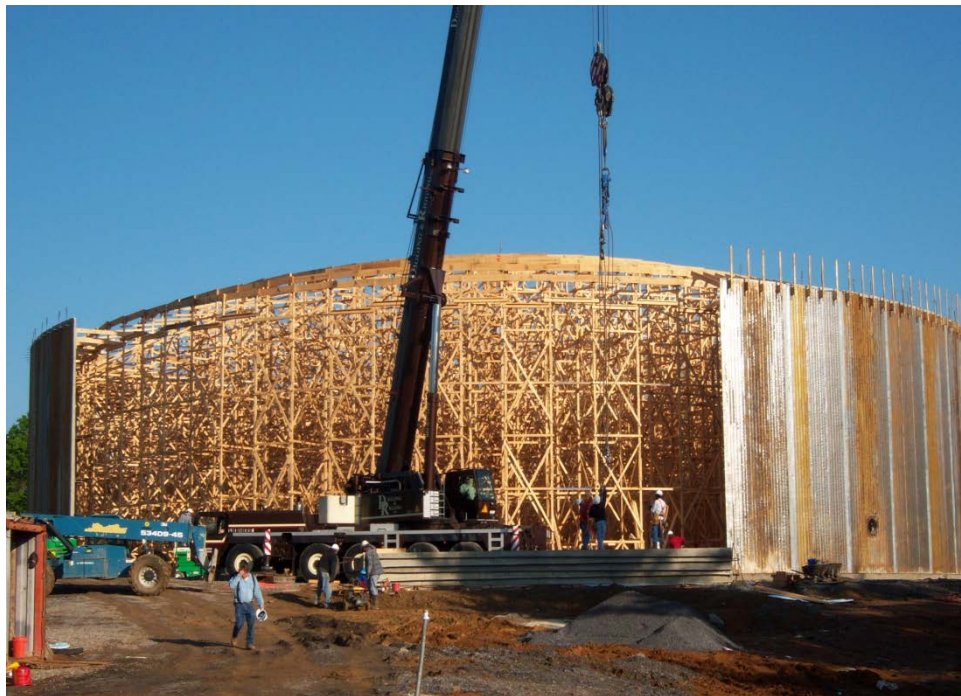
FIGURE 1. HELLANE PARK TANK UNDER CONSTRUCTION
