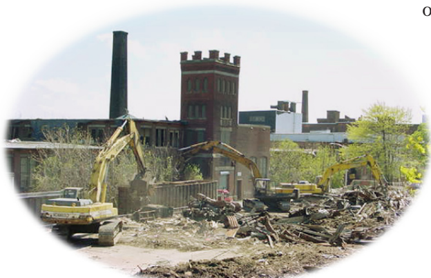
Demolition underway before construction of the new facility.
