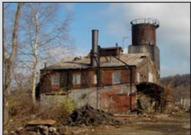
The Firth Sterling steel mill before redevelopment.
