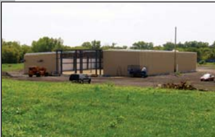
New lumber store under construction at the former NWSW mill.
