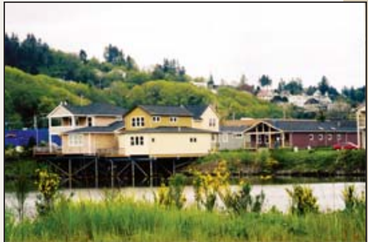
The Mill Pond Village development along the Columbia River.
