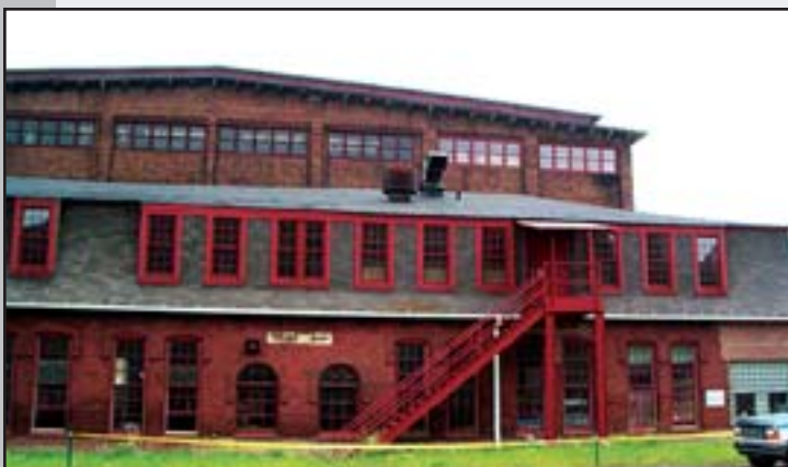
The Cambria Iron Works carpenter shop building after renovation.
