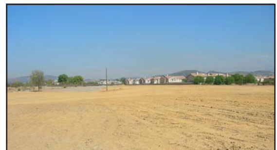
This 5-acre cap in the City of Orange was constructed over a former landfill to make way for greenspace, parking and planned development at Grijalva Park.
