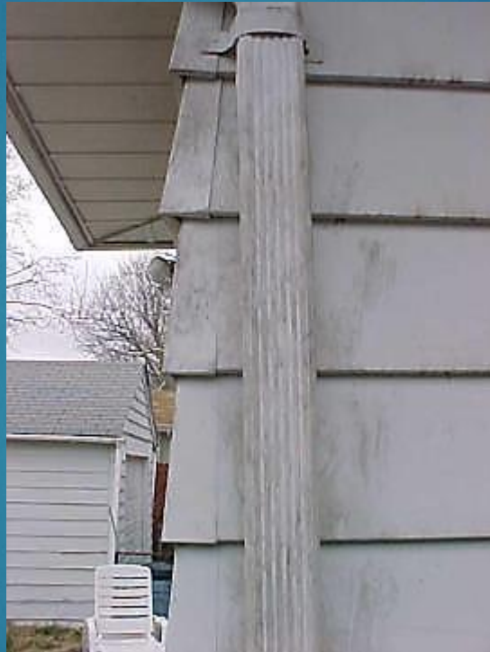
Smudge marks on downspout
