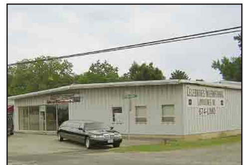
Commercial activity is restored on the Midlothian Corridor.
