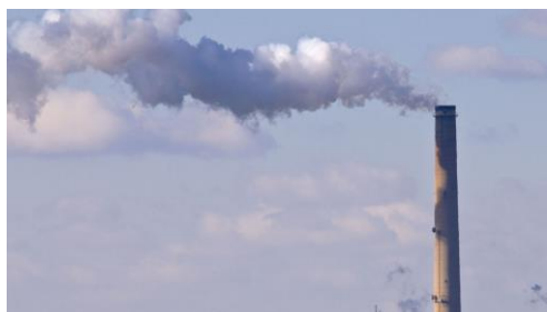
A smokestack at a coal-fired power plant. (EPA photo)
