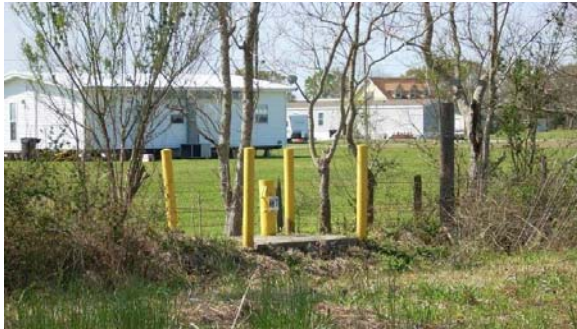
Monitoring well MW-7 at the remediated PAB Oil site. (EPA OIG photo)
