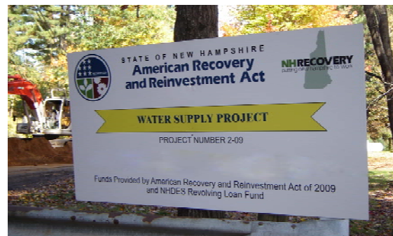
Sign identifying a water project in New Hampshire funded by the Recovery Act. (EPA OIG photo)
