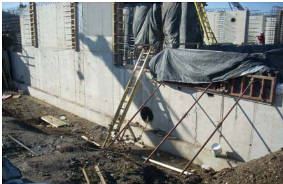
Wastewater treatment facility under construction in the City of Newark, Ohio. (EPA OIG photo)
