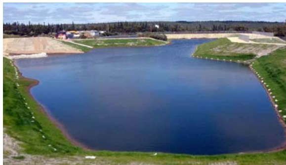
New Stuyahok, Alaska, sewage lagoon constructed by the Alaska Native Tribal Health Consortium and partially funded by interagency agreement DW 75-95754001. (Photo from Alaska Native Tribal Health Consortium website)
