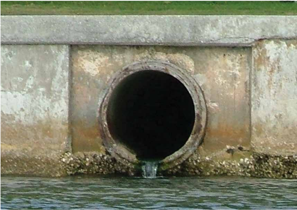
Stormwater discharged through pipes delivers pollution to the Bay. (New College)
