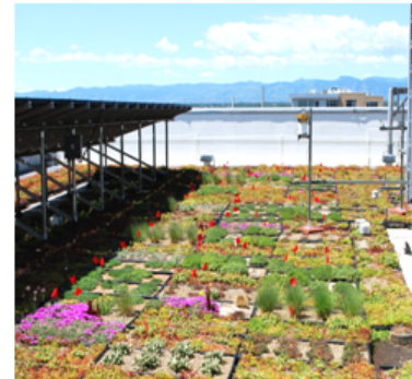
The EPA Region 8 Headquarters' green roof with study plots and instrumentation. The solar panels provide beneficial shade during hot weather. Photo: EPA Region 8.
