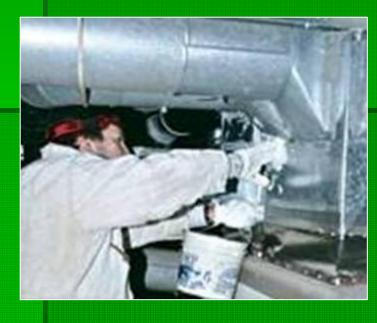
Critical Duct Sealing directly above furnace where majority of heat escapes from ducts
