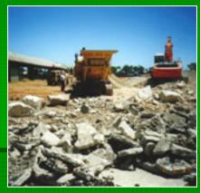
Crushed concrete as aggregate in new concrete
