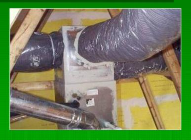
Throughout the U.S, duct leakage typically wastes 10% - 30% of the heating or cooling energy purchased by a homeowner
