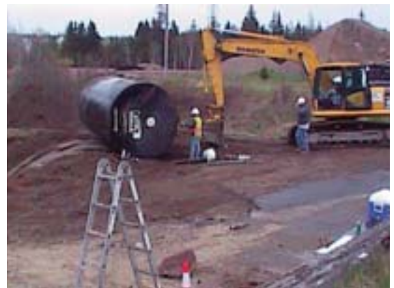
Tank Removal Activities at the Sipiyak Corner Store Property
