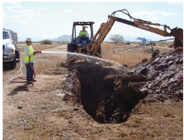
Cleanup Activities at the Feedlot Property
