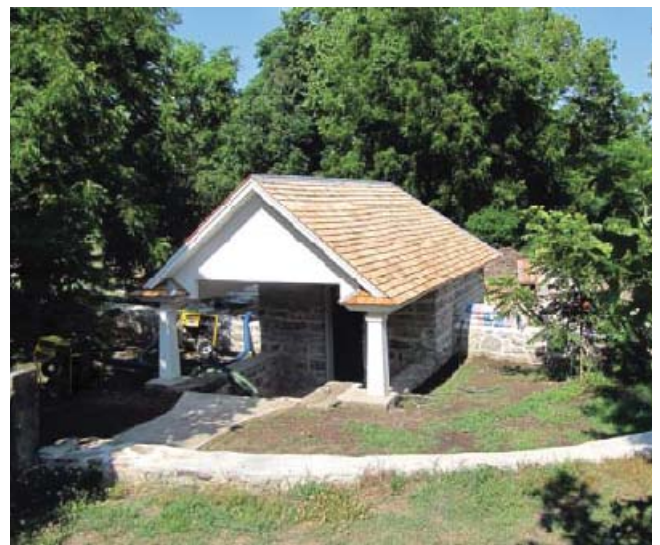
The Springhouse on the Saline Courthouse National Park Property During Redevelopment
