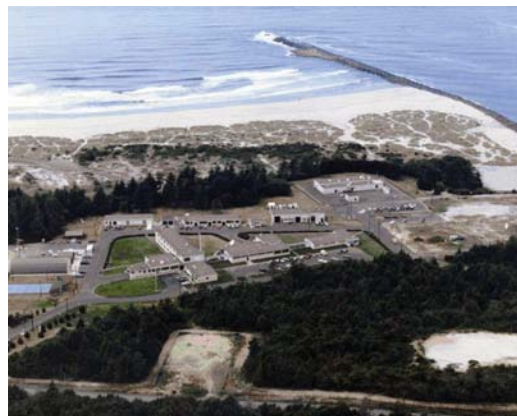
Aerial View of Coos Head Property
