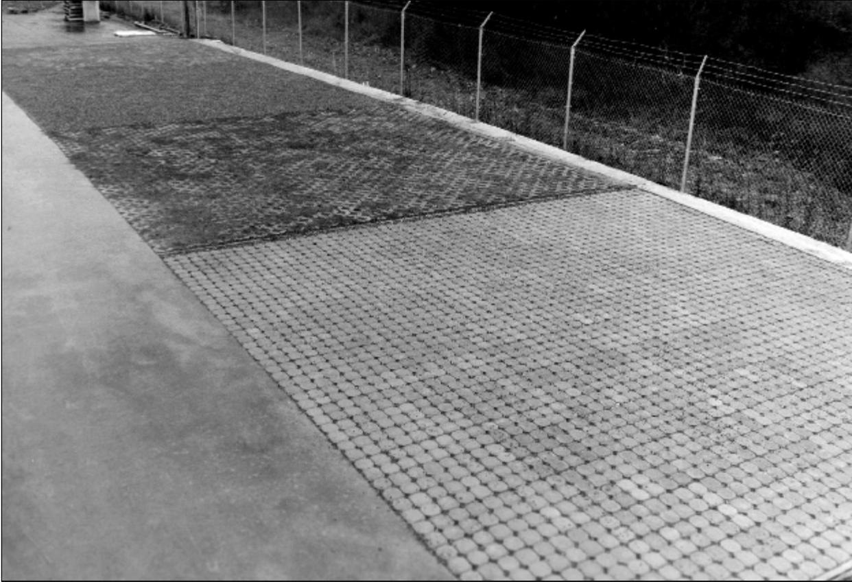
**Figure 5.3: Photo showing several types of pervious modular pavement installations.**
