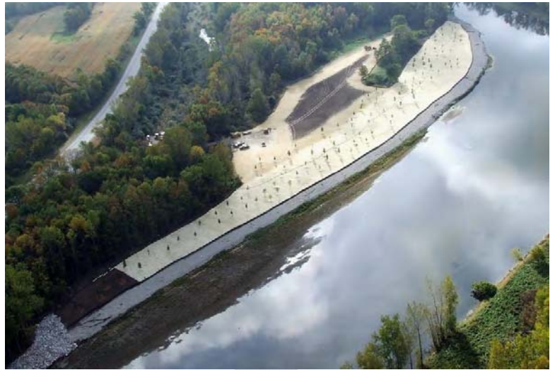
Floodplain and bank soil removal – About 30,000 cubic yards of soil and 300 mature trees were removed.
