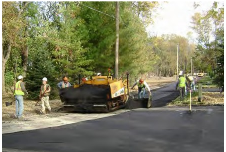
Covering road with new asphalt.
