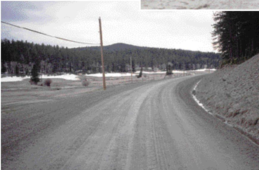
Remarkable difference in these two roads that carry similar volumes of traffic. They are located in the same region of the country and the photos were taken on the same day. The major difference is drainage. The upper photo shows a well-drained road while the lower photo shows a poorly maintained ditch that resulted in a poor performance.
