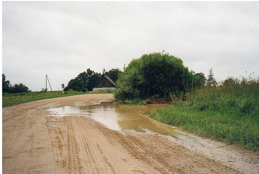
Lack of a roadside ditch has caused major drainage problems on this road. (Courtesy of Road Research Ministry of Roads/Transportation, Sweden)
