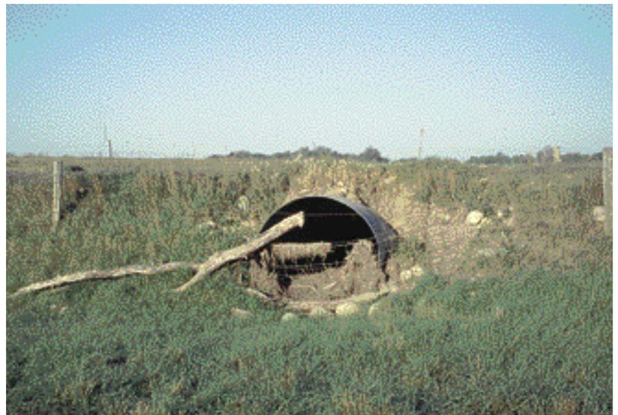
This road could fail if debris is not cleared before the next heavy rain.
