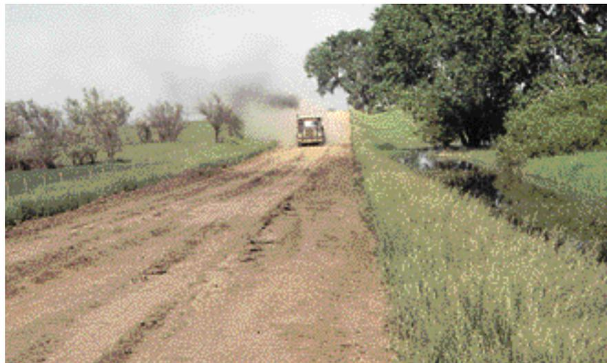
This road has been badly damaged from a heavy haul. It would be useless to begin hauling and placing fresh gravel until the entire roadway has been reshaped.
