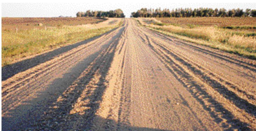
These two roads show remarkable contrast in surface condition due to the quality of gravel. They carry virtually the same volume and type of traffic in an agricultural community. The top photo shows a good surface gravel with a nice blend of material, particularly some plastic fines which keep the surface tightly bound. The bottom photo shows a road surface that has too much stone and sand in proportion to the fine material. Consequently, the gravel remains loose and is hard to maintain.
