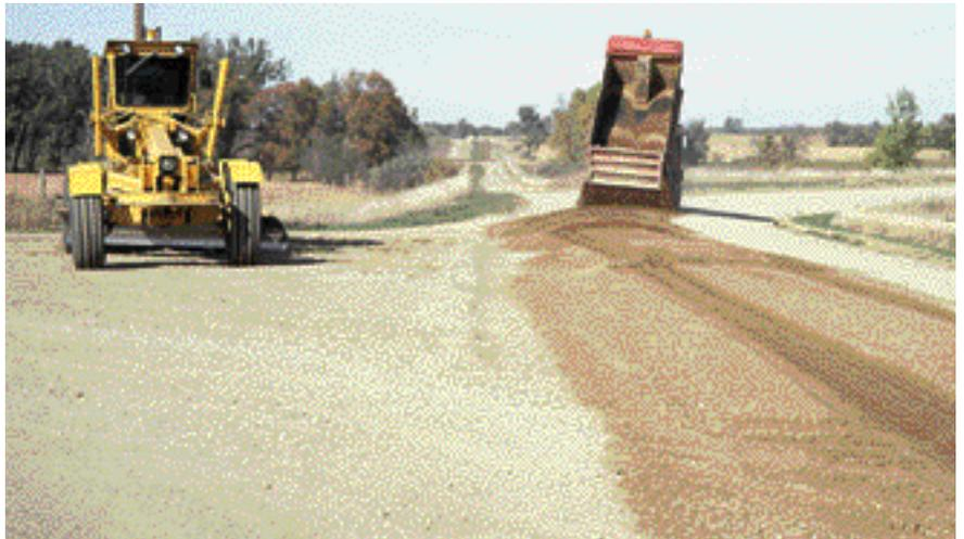
Once hauling begins, it is wise to have a motorgrader present to process and place the gravel immediately. The skill of the truck drivers can really make a regravelling operation work smoothly. When drivers are able to dump the load evenly and within the correct length that was marked, the grader operator's job becomes much easier.
