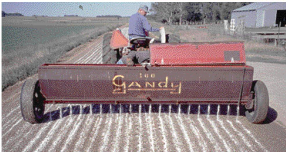
A very effective, yet simple method of applying flake Chloride accurately with an old farm fertilizer spreader. These machines can be calibrated with great accuracy. Quick cleanup afterward is important since Chloride is corrosive to equipment. Once it is bound in the gravel, corrosive effect on vehicles is very low.
