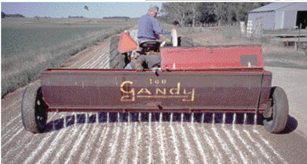
A very effective, yet simple method of applying flake Chloride accurately with an old farm fertilizer spreader. These machines can be calibrated with great accuracy. Quick cleanup afterward is important since Chloride is corrosive to equipment. Once it is bound in the gravel, corrosive effect on vehicles is very low.
