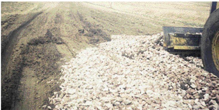
The dozer attachment allows this operator to push a load of rocks into a frost boil with the grader. Without this option, a loader would likely have to be brought to the job.
