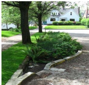
Vegetated curb extensions used to decrease stormwater runoff as part of a “green reserve” project. (EPA photo)
