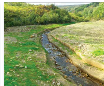
Figure 3. The new Slate Creek stream channel, shortly after project completion.
