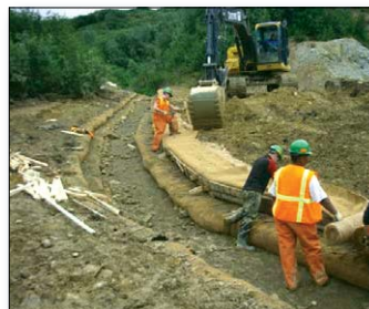
Figure 2. A new section of the Slate Creek stream channel, under construction.
