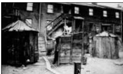
Privy vaults and water pump are located side-by-side in this Pittsburgh neighborhood, circa 1909.
