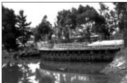
San Francisco's Islais Creek Transport/Storage Facility stores and conveys flow to the Southeast Plant. With a 600-foot overflow weir and 45 mgd storage capacity, this facility reduced combined sewer overflows from 40 to the allowable 10 per year.
