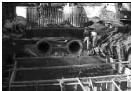
CSO separation project underway in Louisville, Kentucky.
