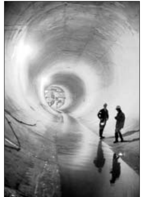
Chicago had one of the nation's earliest large-scale CSO control programs. As of 2001, Chicago's Tunnel and Reservoir Project (TARP) has cumulatively captured 565 billion gallons of combined sewage that would otherwise have flowed to area receiving waters.
