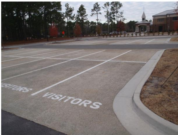
**Figure 12. Pervious Concrete Parking Stalls.**
