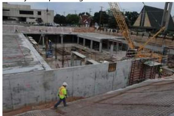
*Cast-in-place Concrete Tank*
