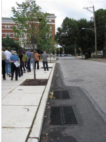
**Figure 11. Tree Box Using Grate Inlets in Street.**
