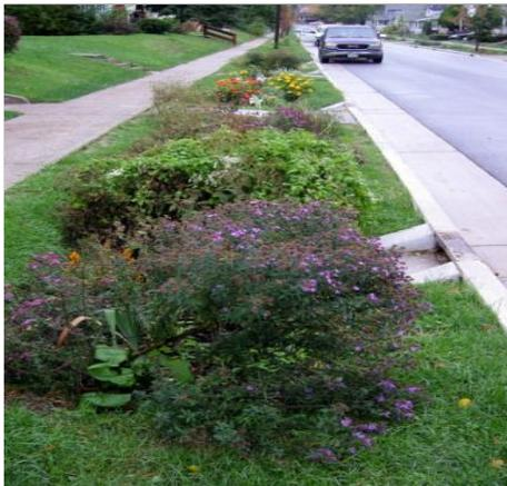
**Figure 7. Bioretention Incorporated into a Right-of-Way.**
