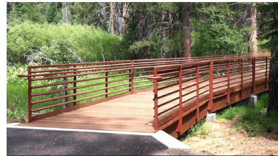
The boardwalk trail was constructed above the wetlands and strategically meanders to eliminate impacts on water quality and existing trees.
