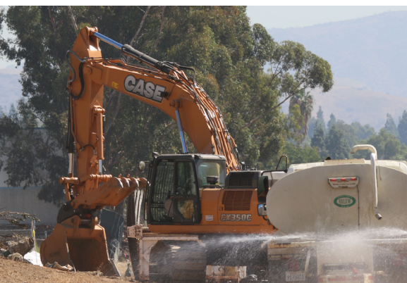
Soil remediation is underway along this 1-mile corridor in Brea that will be converted to a linear park featuring bicycle and pedestrian trails.
