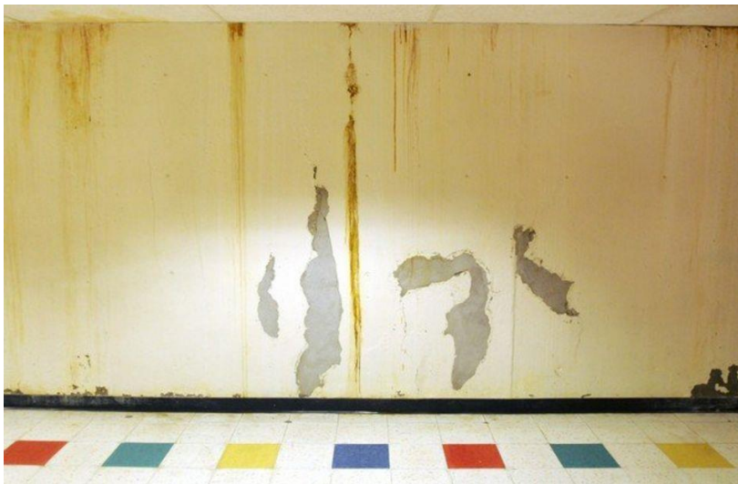
Figure 3. Peeling wall paint and water-stained walls in the tunnel walkway (photo by Mark Murray from a February 9, 2012 article in the Republican).
