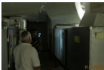
HIA project team surveying the HVAC systems
