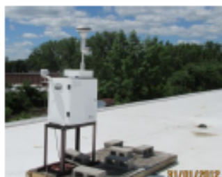
Air monitor on roof of school
