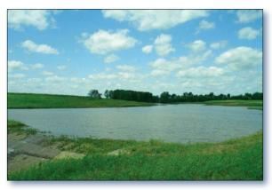
Figure 2. Example of a sediment pond constructed along a tributary stream in an agricultural watershed. The pond is designed to remove suspended and soluble nonpoint source pollutants.
