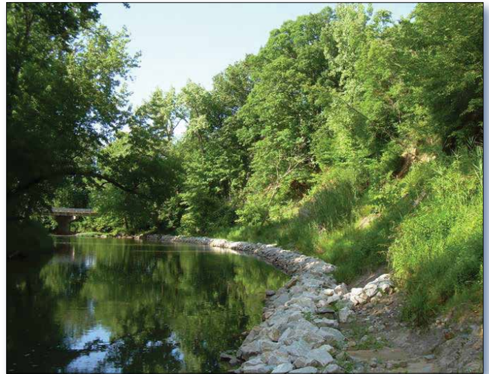
Figure 2. A CWA section 319-funded streambank stabilization project on the North Fork Vermilion River.
