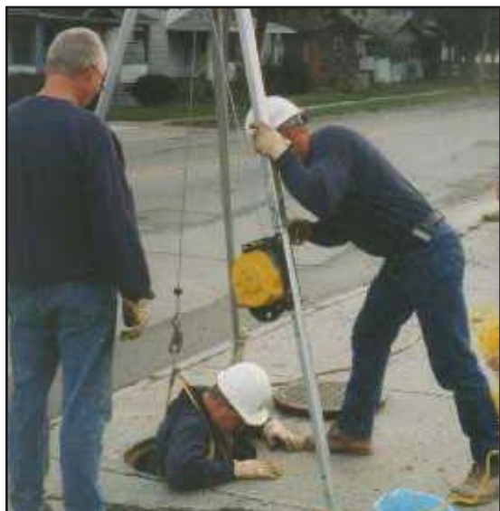
Trackdown sampling involves sampling water in local sewer systems for contaminants such as PCBs. Photo Credit: USEPA
