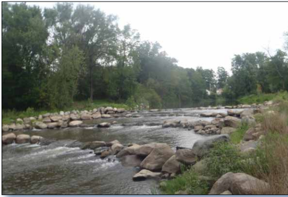
Figure 2. After the Nashville Dam was removed, Michigan DNR installed a four-tiered rock ramp.
