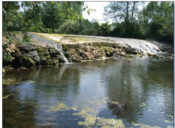
Figure 1. The Nashville Dam trapped sediment behind it, leading to low DO levels in the Thornapple River.
