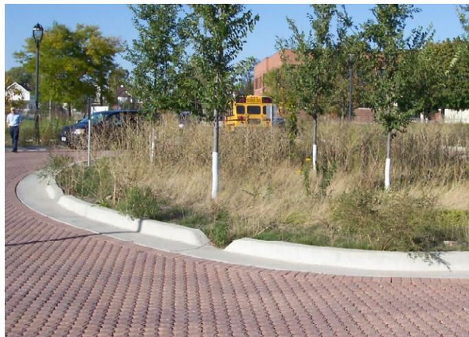
Above: A rain garden in a roundabout designed to capture and infiltrate stormwater in Milwaukee, WI. Left: Rendering of a curb bumpout along a residential street. Below: Cut-away of a curb bumpout with permeable pavers on sidewalk.
