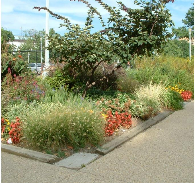
*Above: Rain gardens allow rain and snowmelt to seep naturally into the ground while also providing visually appealing landscaping. Below left: Rain gardens work equally well in residential areas. Below right: A bioretention cell filters rainwater in a shopping center parking lot.*
