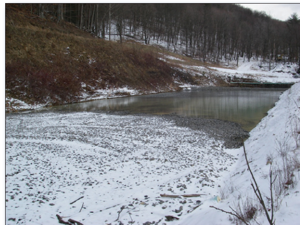
Figure 1. This limestone pond treats AMD in the Miller Run watershed.
