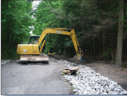
Figure 2. Partners added limestone rock to roadside ditches on the State Game Lands #67 access road to provide passive treatment for runoff.
