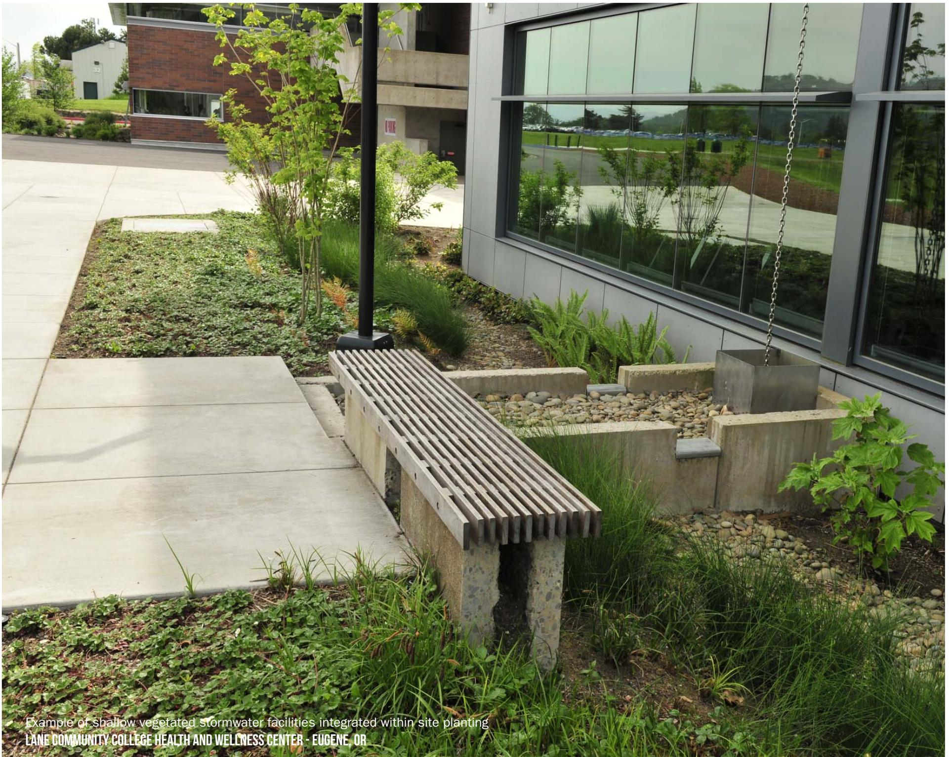
Example of shallow vegetated stormwater facilities integrated within site planting
