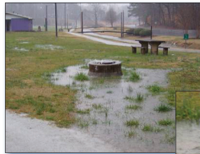
Figures 1 and 2. Manholes like this one in a park adjacent to Cane Creek would routinely overflow and spill raw sewage during rain events.
