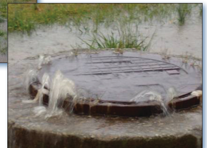
Figures 1 and 2. Manholes like this one in a park adjacent to Cane Creek would routinely overflow and spill raw sewage during rain events.
