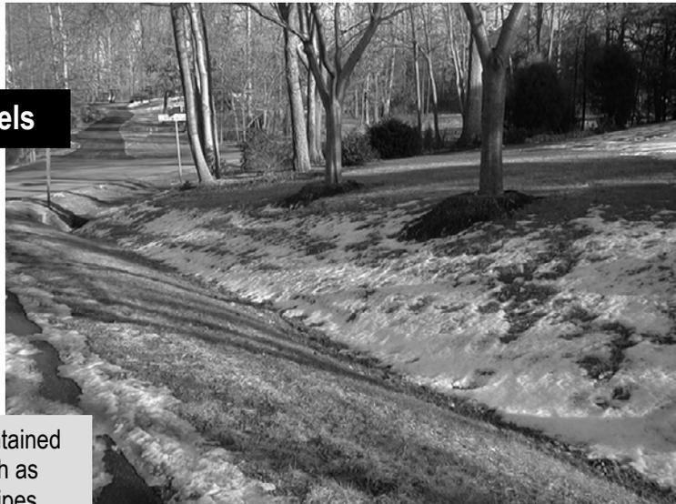
Natural drainage courses can be maintained by using grass-lined channels as much as possible instead of concrete canals, pipes, and gutters.
