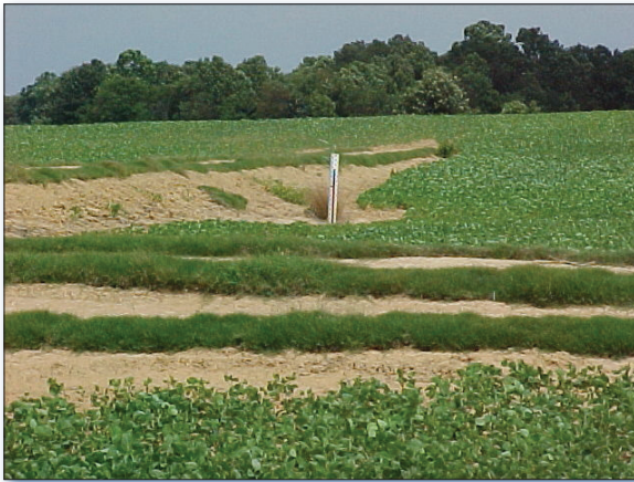
Figure 2. Water and sediment control basins such as this one prevent bank and gully erosion on farmland. The runoff water is temporarily stored behind the berm, eliminating its erosive capabilities further down slope. The ponded water slowly flows out through an inlet riser pipe (center) to an underground tile drainage network.
