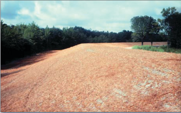
Figure 2. Example of a dike, or earth embankment.
