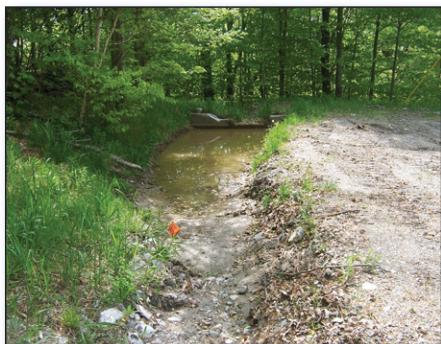
Figure 2. Sugarbush Resort built treatment swales to control stormwater flow in ditches along private roads in the Sugarbush Village area.
