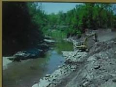
In the spring of 2011, the steep, eroded streambank was reshaped to a more gentle slope, designed to minimize erosion, prevent bank collapse and allow riparian vegetation to regrow.
