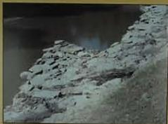
Rock was placed at the toe of the slope, and in the river in rock vanes, designed to deflect flow from the streambank and trap sediment.
