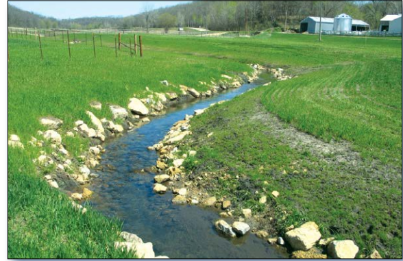
Figure 3. Project partners installed livestock exclusion fencing and restored the stream channel and its natural meanders.
