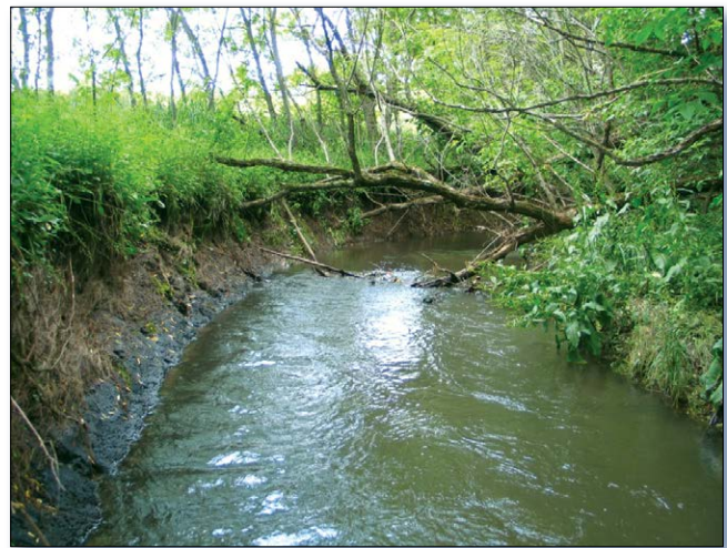
Figure 1. Before restoration, German Valley Branch was deeply entrenched and had highly eroding banks.
