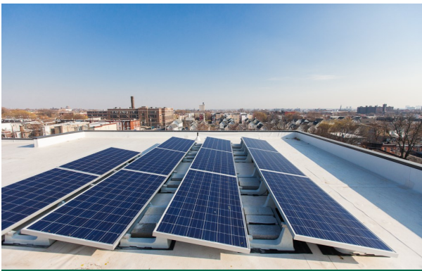
Solar panels on the roof, courtesy of Paul Gargagliano
