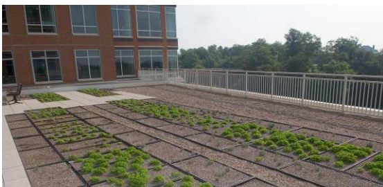
A “green,” stormwater-management roof on an EPA building in Arlington, Virginia (EPA photo).
